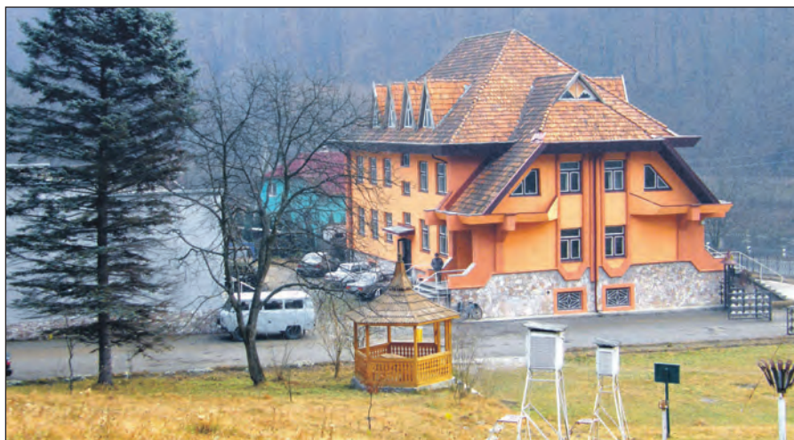
One of the buildings of the Central Office of CBR
